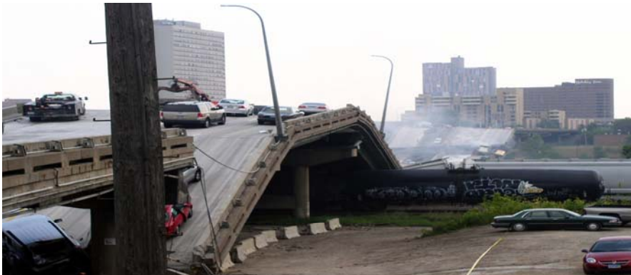
Bridge Image: I-35W Bridge Collapse, Minneapolis, MN, August 1, 2007. Released into the public domain by its author, Tom Ruen at the English Wikipedia project.
